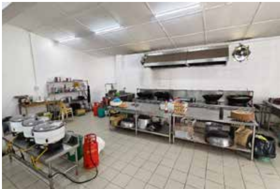
New Canteen Kitchen area
