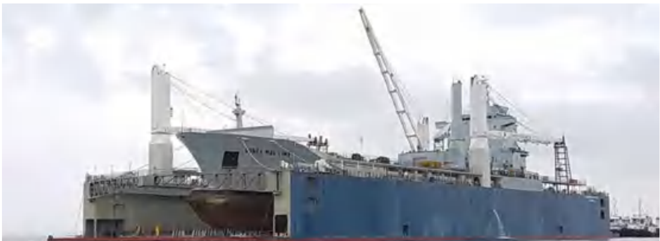
160m floating dock in empowering marine works
